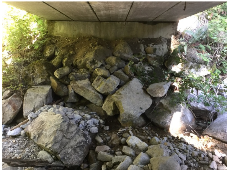
Right Bank Abutment when facing downstream
