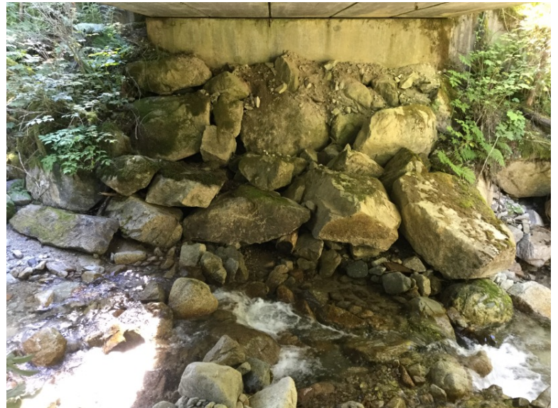
Left Bank Abutment when facing downstream
